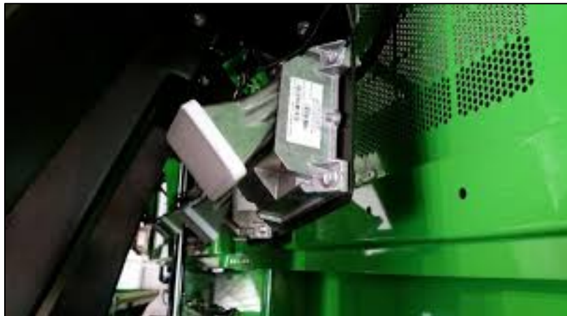
Figure 2. Microwave John Deere Mass Flow Sensor on backside of air ducts
